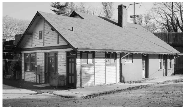
The Cynwyd Train Station as it looks today. View is of the west side facing Conshohocken State Road
